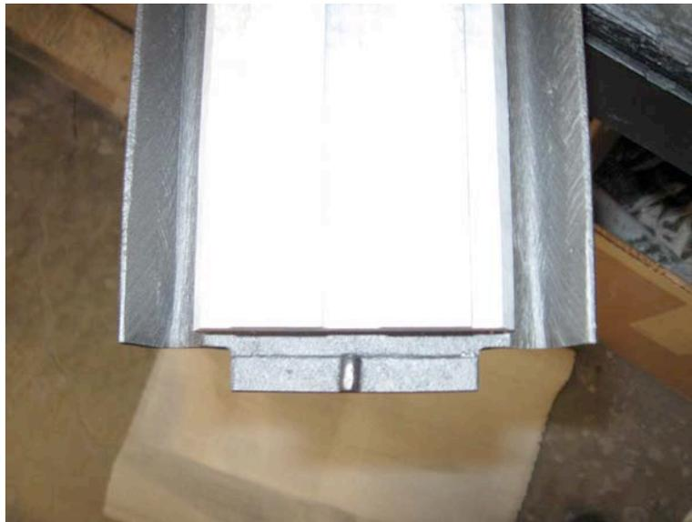
12. Now install the stone and corner cast into the stove by placing the bottom into position first. Once the bottom edge is in properly you should be able to swing the top edge in as you lift up on the top frame for clearance. You will need to position the rope around the corner cast to get it in place.
