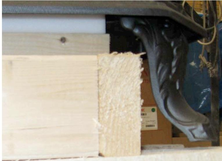
4. Tie a rope around the stove about two inches below the top cast lip. You may also use an adjustable nylon strap. **This will be the only thing holding your stove together while you perform the procedure.**
