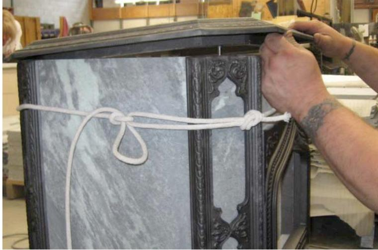
8. Pull the corner out past the edge of the top frame then lift up on the corner. Lift it up and out of the base of the stove. The stone may stay in place as the cast is removed or it may want to fall out along with it.
